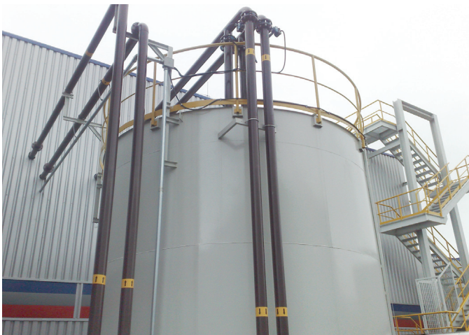
TANQUE DE AVARIAS E DESCARTES TANK FOR DAMAGED AND DISCHARGED MATERIALS
